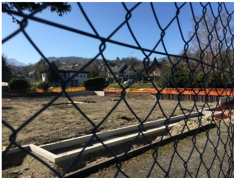
Travaux courts couverts TC La Motte Servolex
